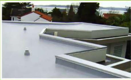
ROOF SLABS & SCREEDS
