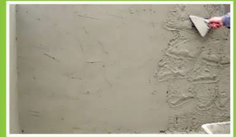
INTERNAL & EXTERNAL PLASTERING
