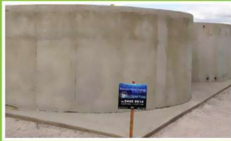
WATER TANKS & WATER RETAINING STRUCTURES
